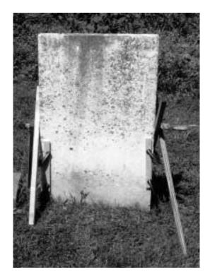
After the repair has been made, securing the marker is imperative. The use of clamps, wooden braces and shims assures the headstone is not touched by the metal clamps, and also prevents the headstone from moving while the repair treatment cures.
